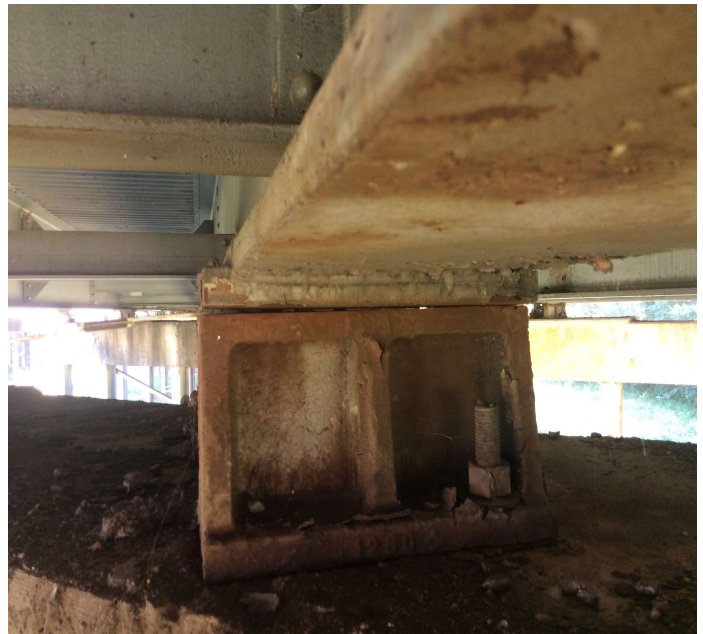
PHOTO 2 Description Bent 5 fixed bearing 3 has up to 3/8" gap between the bearing and sole plate. bearing 4 has a gap also.
