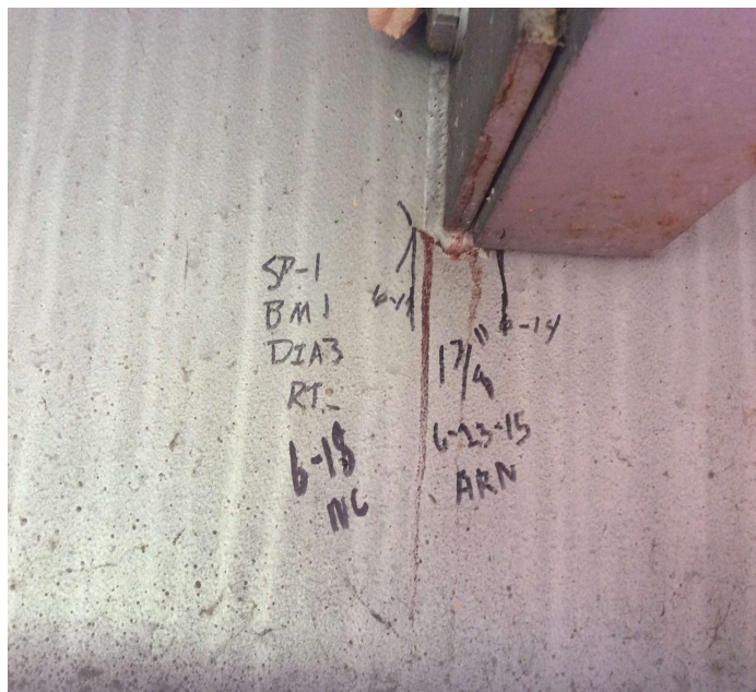
PHOTO 4 Description Span 1 girder 1 diaphragm 3 crack in web.
