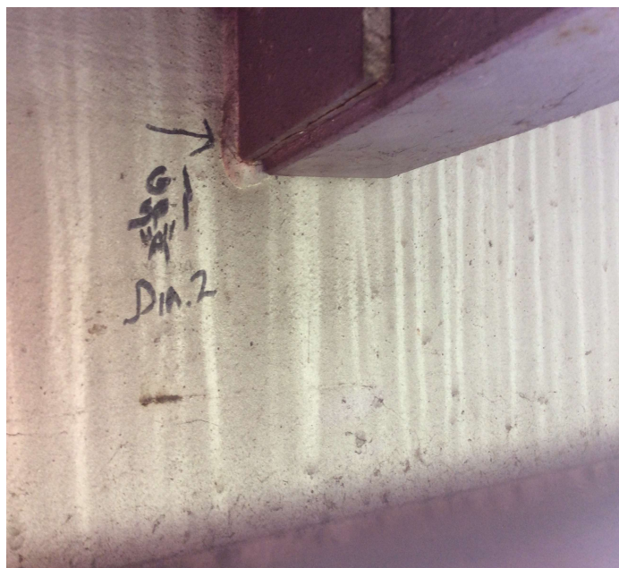
PHOTO 3 Description Span 1 girder 1 diaphragm 2 crack in toe of weld
