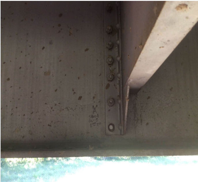
PHOTO 1 Description Span 4 girder 5 missing bolt.
