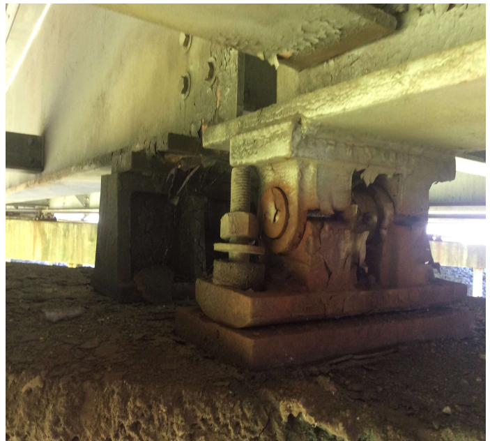
PHOTO 2 Description Bent 4 moveable bearing 4 has movement under traffic impact.
