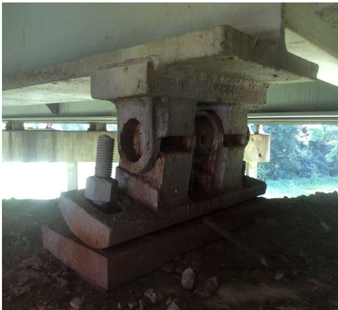
PHOTO 1 Description Bearing pin working out.
