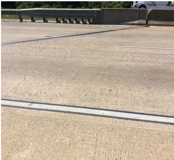
PHOTO 1 Description Large transverse cracks in right lane.
