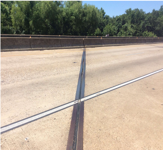
PHOTO 1 Description Bent 5 joint has lost adhesion in both lanes.
