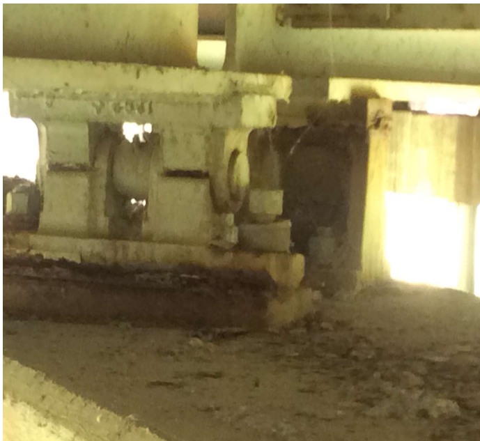
PHOTO 1 Description Most bearings have heavy pack rust build up.
