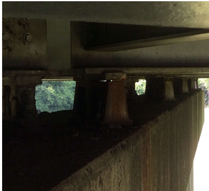
PHOTO 1 Description Gap between bearing and sole plate.
