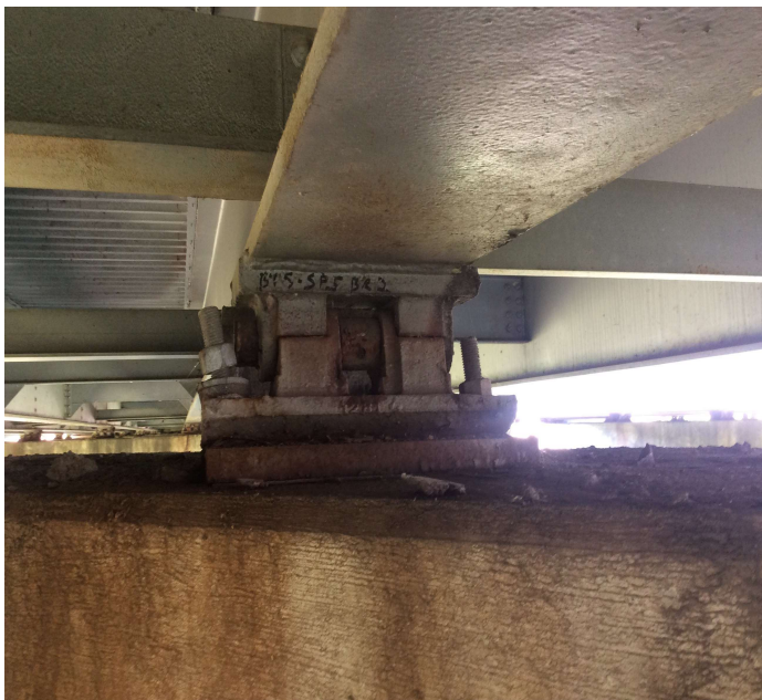
PHOTO 3 Description Bent 5 moveable bearing 3 pin is working out.
