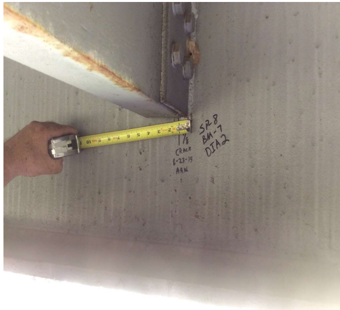
PHOTO 1 Description Span 8 beam 7 diaphragm 2 has a 7/8 inch crack in the web
