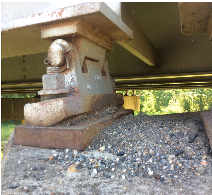
PHOTO 3 Description Bent 4 bearing 1 ahead side has pack rust. Typical for moveable bearings.
