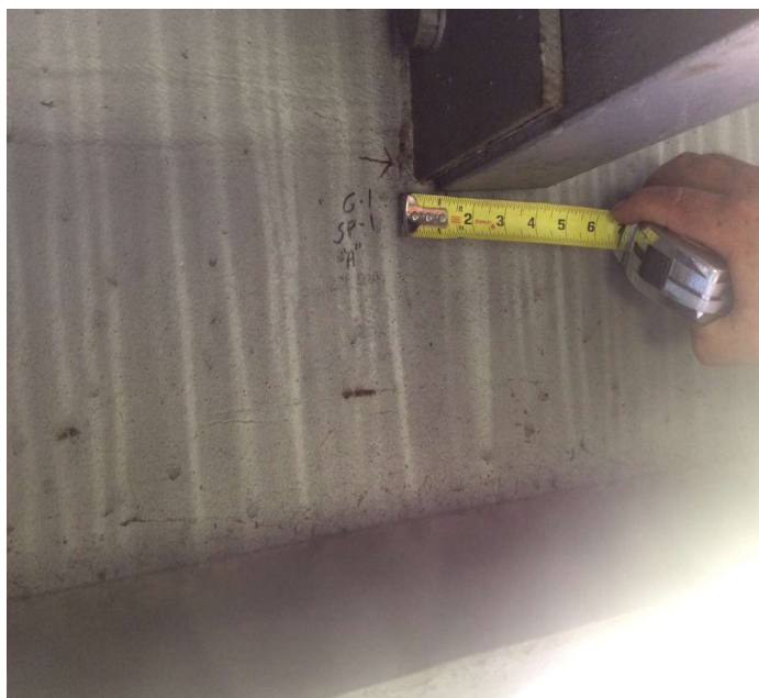
PHOTO 7 Description Girder 1 span 1 diaphragm 2 has a 1 inch crack in the web
